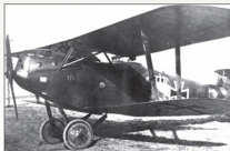
Hannover Cl.II 13189/17 from Bavarian FA 287b is shown here in early 1918. Note the additional tailplane bracing struts ( D9 ), pilot's rear view mirror ( 679 ) and the Bavarian blue and white diamond wappen (heraldic shield) on the fuselage. The weight table 78 is faintly visible under the pilot's cockpit. It should be noted that we are not 100% certain of the wording of the weight table. See pages 24 & 28 for comments on the dark appearance of the underside of the fuselage.
