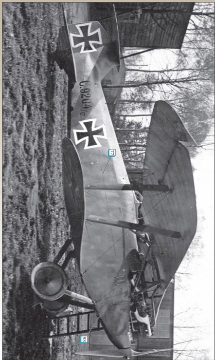
Hanover C.II 9204/17 is one of the very first at-rocket delivered from the initial production batch ordered in August 1917 (numbers 9200/17 to 9299/17). Although not obvious in this photo, another image reveals the fuselage is painted in large irregular 'lozenge' camouflage patches. Note the white(?) exhaust manifolds, fuselage datum line 77 , early production alleron and the lack of wing rigging buttons. Compare the dark appearance of the fuselage underside of 9207/17 with that of 9280/17 below from the same production batch. They would have almost certainly left the factory with the same finish which leads us to believe that the dark effect is simply a dark shadow.
