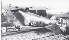
Hannover Cl.II 13189/17 from Bavarian FA 287b is shown here in early 1918. Note the additional tailplane bracing struts ( D9 ), pilot's rear view mirror ( 679 ) and the Bavarian blue and white diamond wappen (heraldic shield) on the fuselage. The weight table 78 is faintly visible under the pilot's cockpit. It should be noted that we are not 100% certain of the wording of the weight table. See pages 24 & 28 for comments on the dark appearance of the underside of the fuselage.
